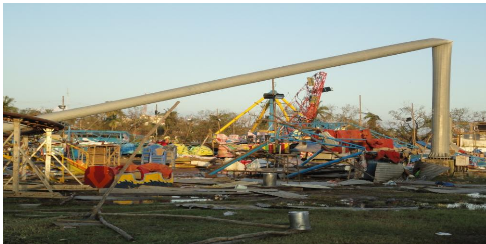
Fig 3 Destroyed circus, Nehru ground, Cuddalore
