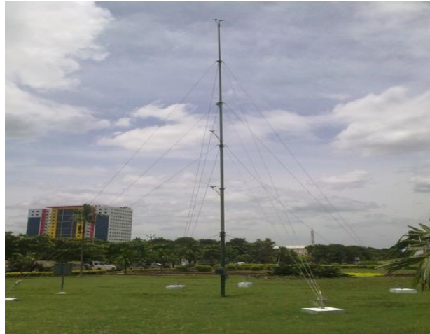
Fig .1 Location of meteorological tower
